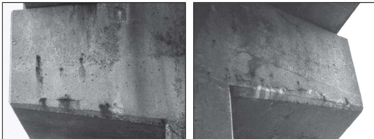
Figure B-11—0.04-in. Width Cracks with Rust Staining in the Cantilevers of the Pier 3 Cap
