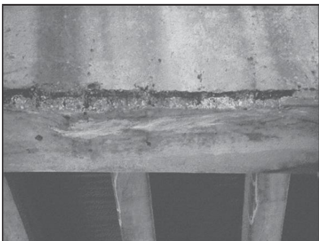
Figure B-10—Spall, Underside of Pier 2 Cap
