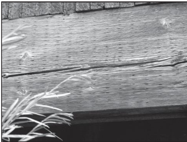
Figure B-2—2-in. Deep Check in Exterior Beam
