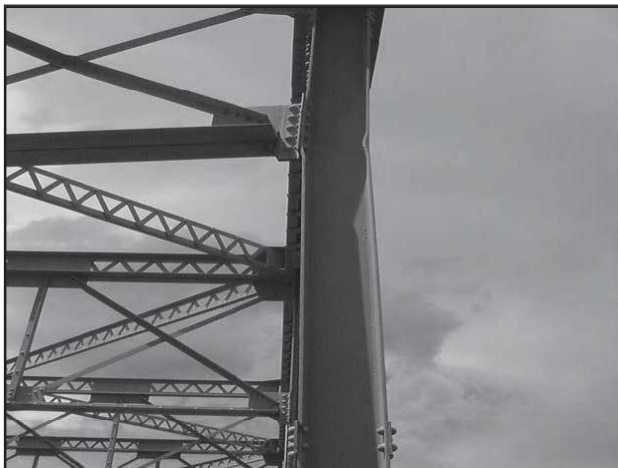
Figure B-15—Sway Bracing Impact Damage in Span 1
