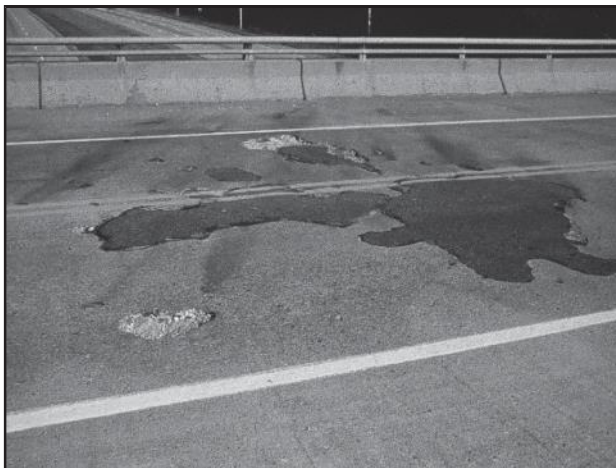
Figure B-7—Spalls and Distressed Patches in Span 2 Deck
