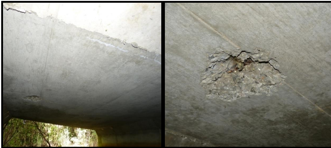
Figure B-28—Spalls with exposed Rebar at Roof Slab.
