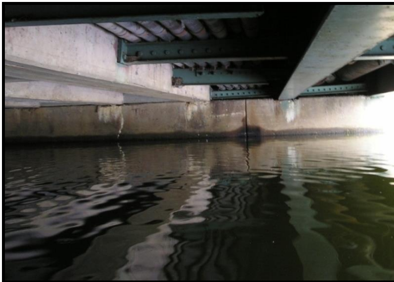
Figure B-25—Typical Efflorescence Staining
