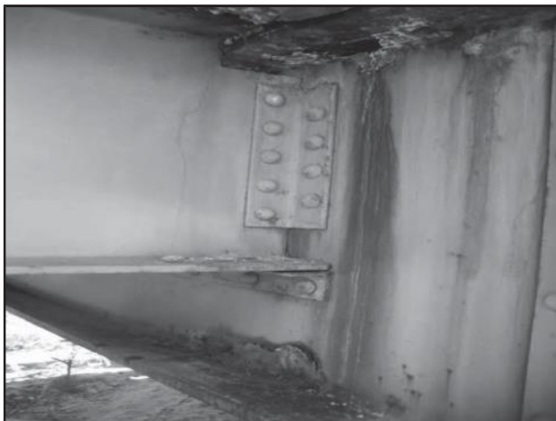
Figure B-17—Corrosion at Floor Beam Ends
