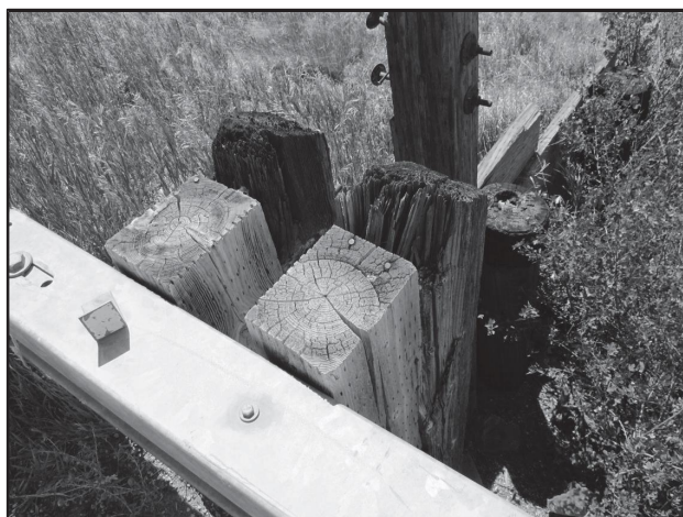
Figure B-5—Decay in Timber Rail Posts
