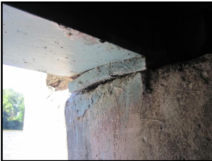
Figure B-23—South Fascia Elastomeric Bearing
