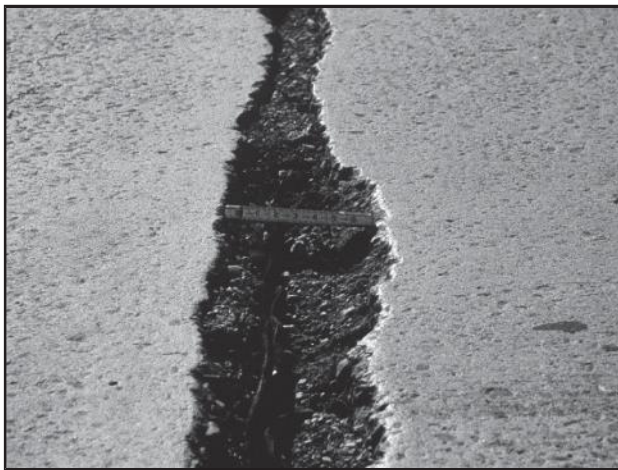
Figure B-9—Deep Spalls in the Deck Adjacent to the Joint Seal at Pier 3
