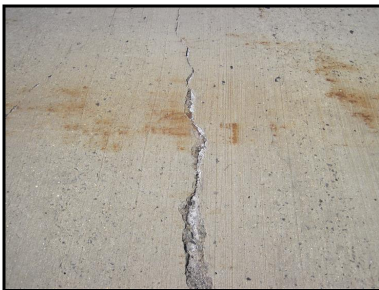
Figure B-21—Wide Transverse Crack on Approach Slab
