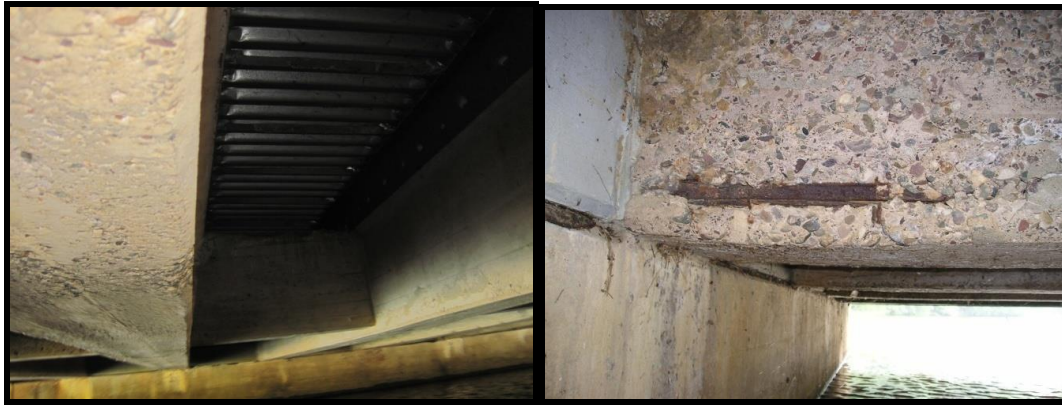
Figure B-24—Typical Concrete Encasement Condition (Left), Localized Spall of Concrete Encasement (Right)
