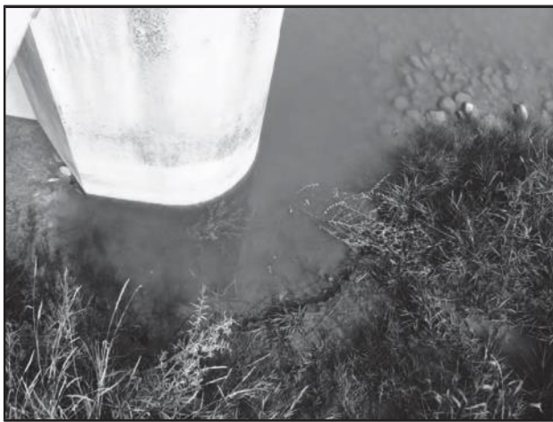
Figure B-19—Scour Hole at the Upstream End of the Pier Wall
